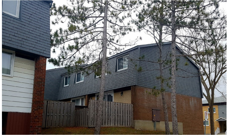
Enviroshingle Installation in Accora Village
